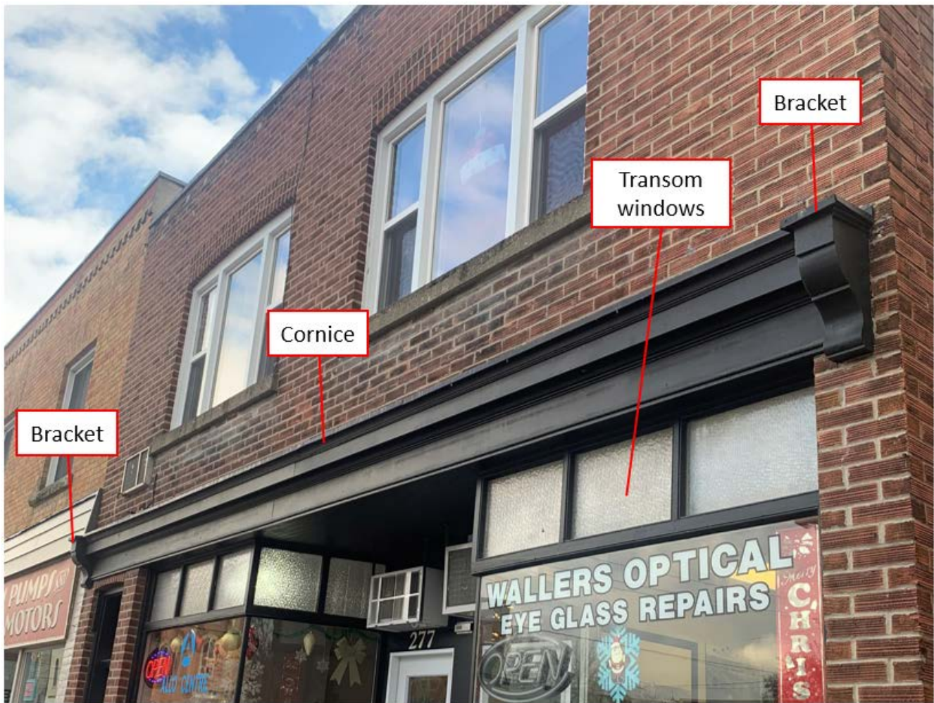
Figure 2: Cornice, brackets, and transom windows of the north (front) facade.
