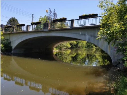
Figures 15 & 16: Vehicular Bridge with BCI rating of 82
