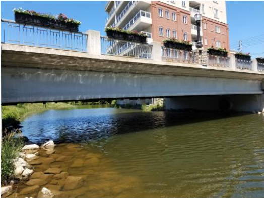
Figures 13 & 14: Vehicular Bridge with BCI rating of 100
