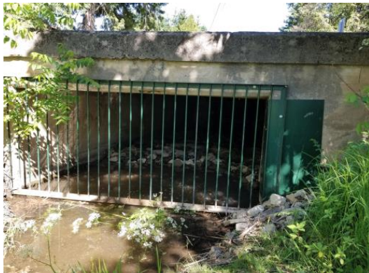
Figures 19 & 20: Culvert with BCI rating of 8
