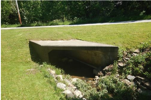
Figures 17 & 18: Culvert with BCI rating of 75
