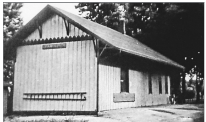
The backside (south side) of the station as seen in the 1940s.
