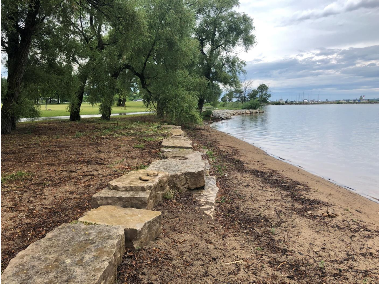
PHOTO 3: willow and other plant life removed
