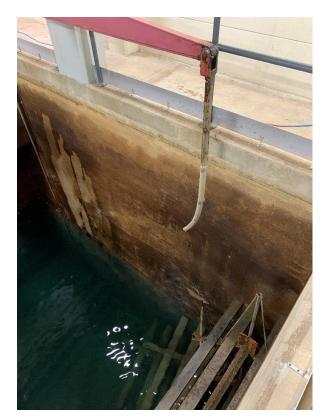
Above left and below: The "paddles" have fallen to the bottom of the tank.
