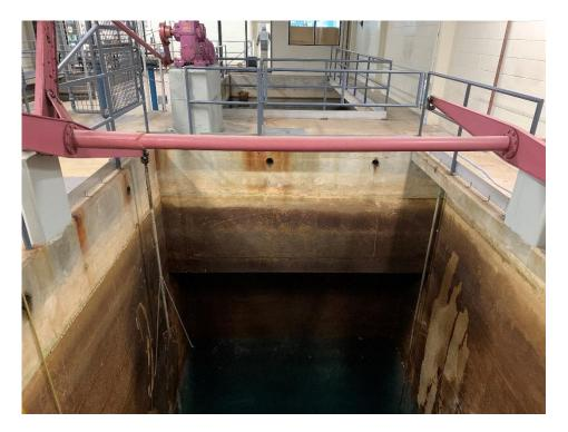
Above: Bowed axle rod. In background, the rusted-through connection of one of the mixing paddle assemblies can be seen suspended from the rod
