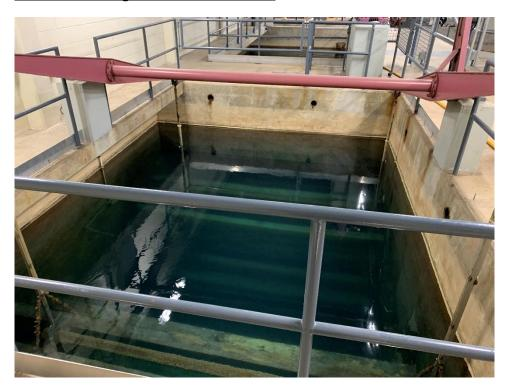
Note the wooden mixing "paddles" suspended from the beams that rock back and forth to repetitively lift and lower each side, thereby mixing the water in the flocculation tank.
