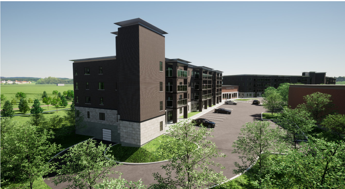
08 - Northern Apt Stair Tower Near Hwy
