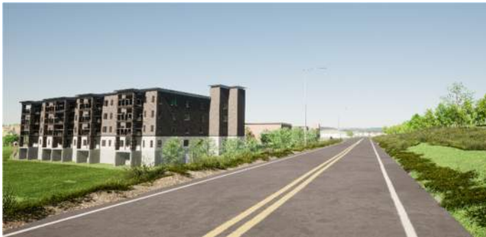
Fig. 3 Residential building with stair tower near the highway - looking west
