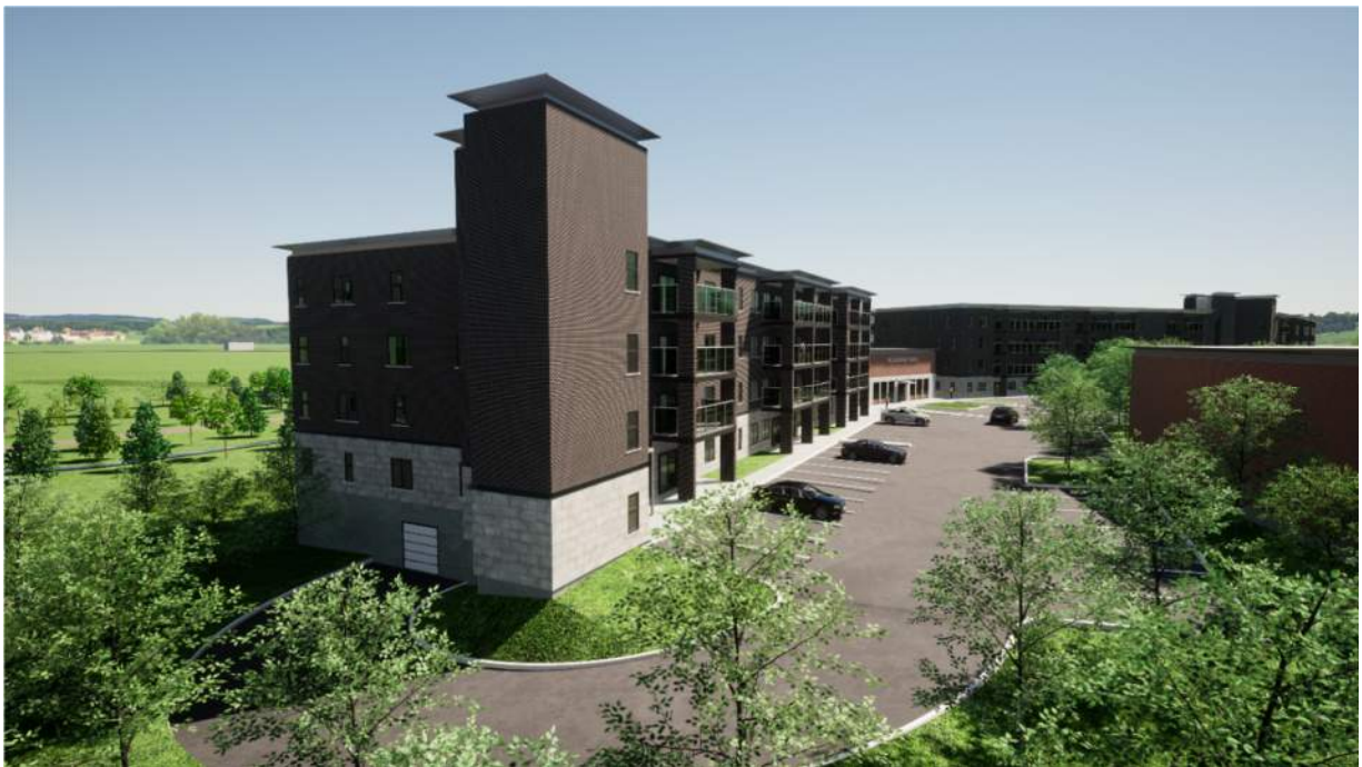
Fig. 5 - Northern Residential Building Near Highway with stair tower.
