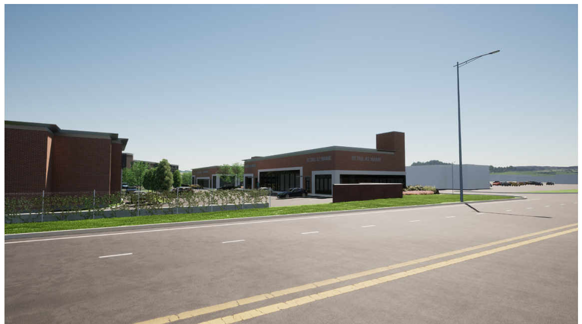
14 - Hwy looking West near New Street Intersection
