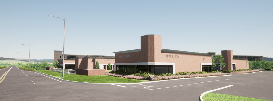
19 - Hwy Travelling East near new street entry 2
