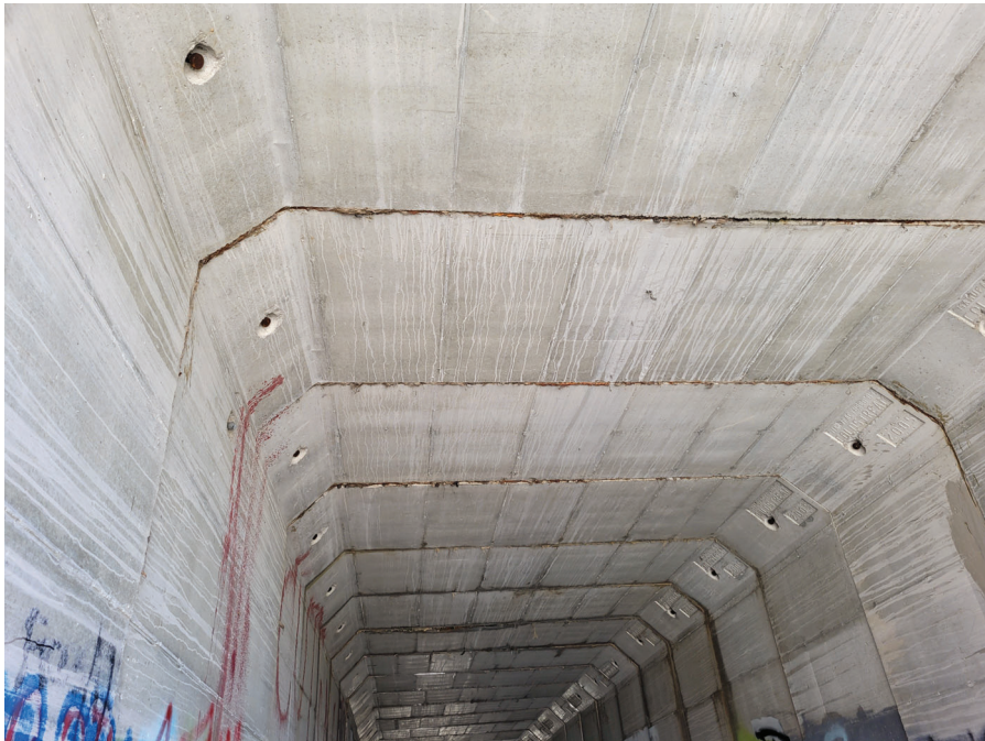
View of soffit.
