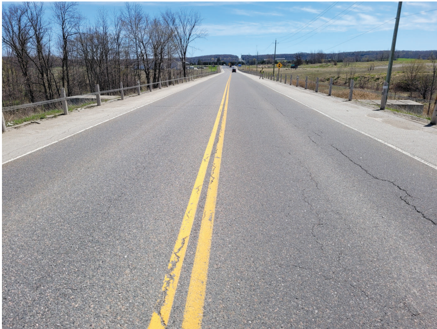
View of structure facing east.
