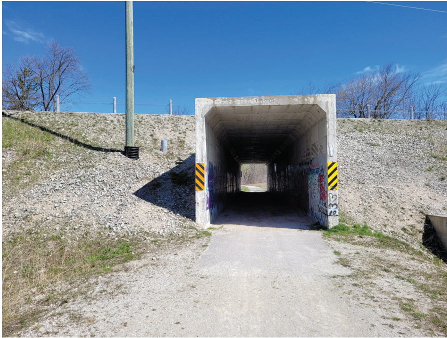
View of structure facing north.
