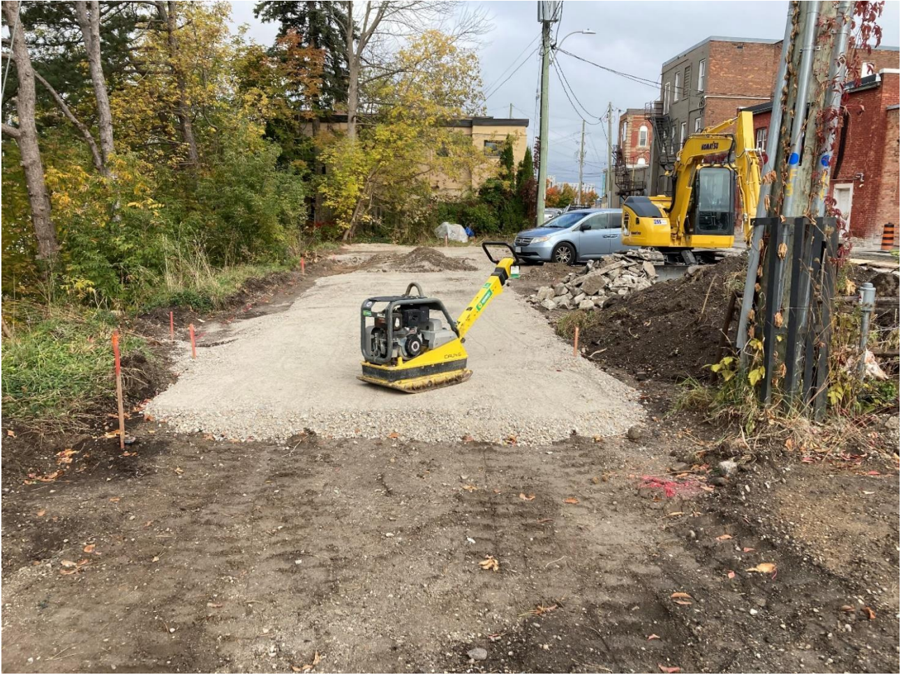
A plate tamper rests atop a bed of gravel where the boardwalk will be installed. Facing North.
