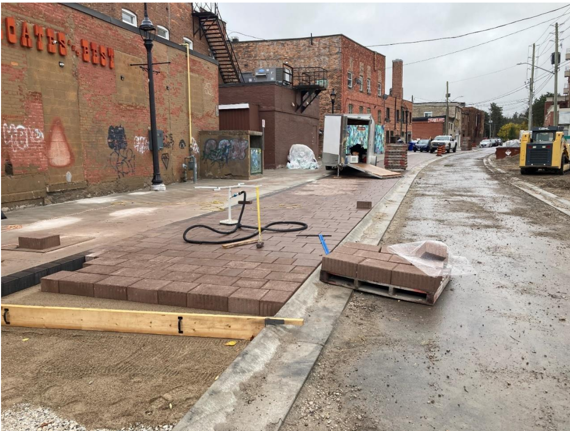
The brick-coloured concrete pavers being installed between the sidewalk and the curb.
