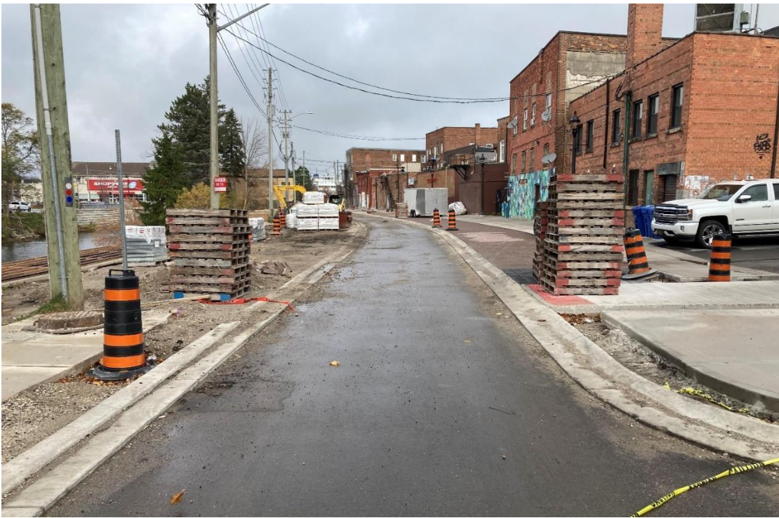
Facing north at the north limit of the bi-directional portion of 1 st Ave East north of 9 th St. New concrete sidewalk and paving stone strip between curb and sidewalk now partially installed.
