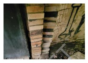
It was also identified that the entrance arches of the inner brick layer, supported by the steel panels, are showing signs of deflection, and some bricks have shifted.
