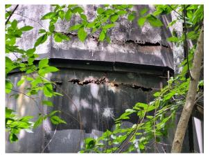
Immediately upon the completion of the on-site assessment, staff from GEI contacted the City to notify staff about structural concerns that needed to be addressed prior to public use of the tower. The most notable concern was considerable corrosion and section loss of the eastern steel panels that support the upper concrete tower and make up the lower portion of the tower.
