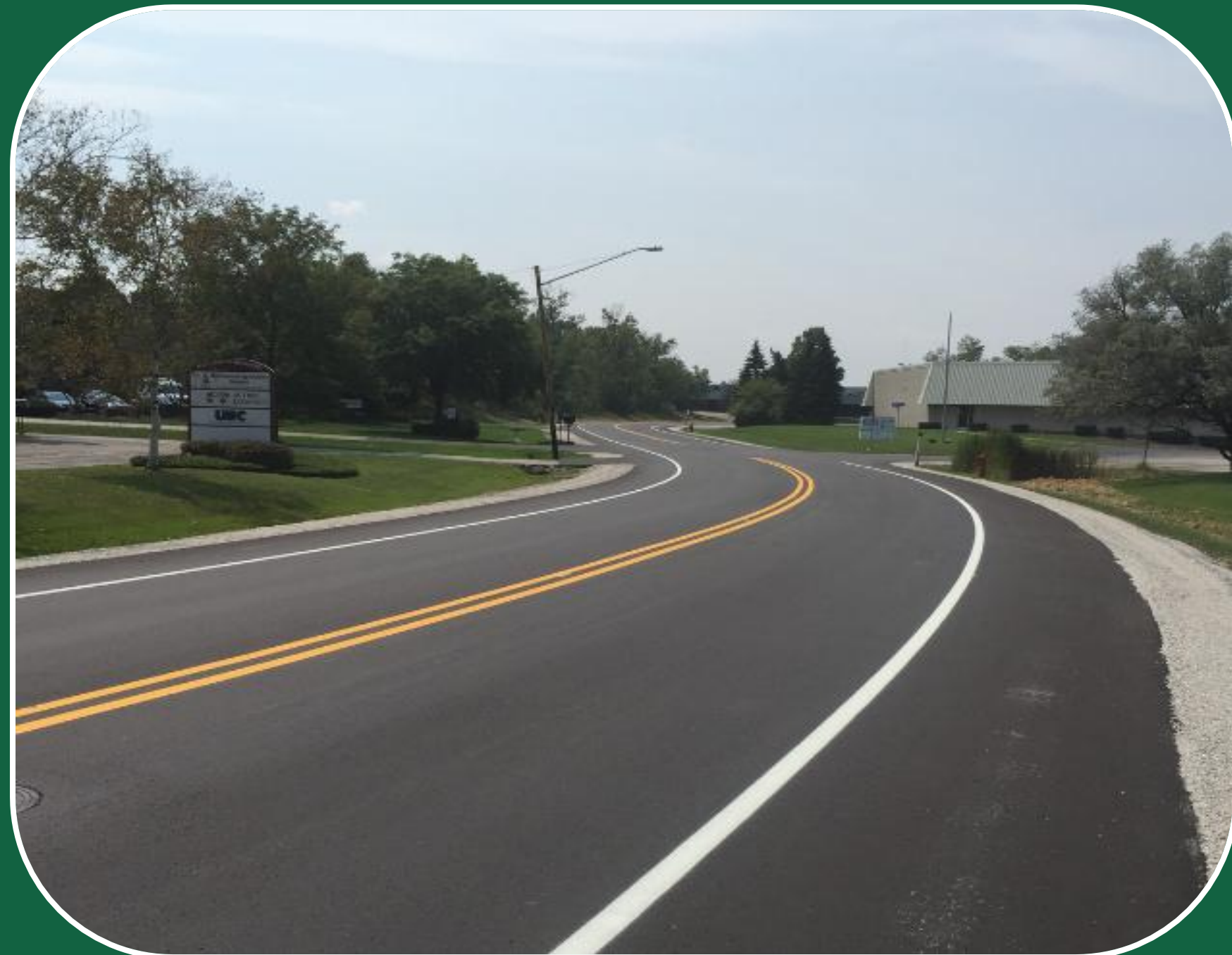
New Eastbound Asphalt Roadway.
