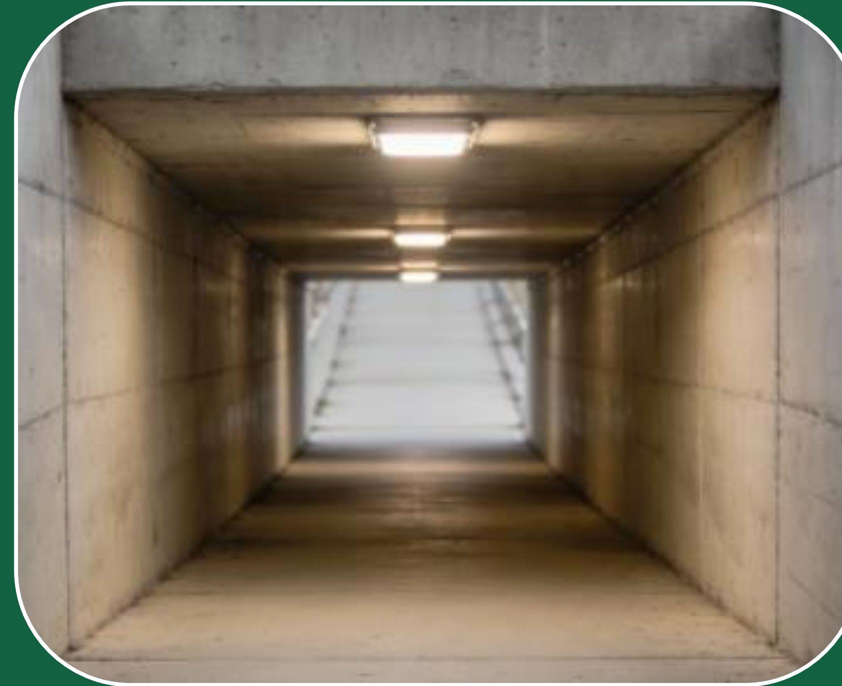
New Lighting Throughout the Tunnel.
