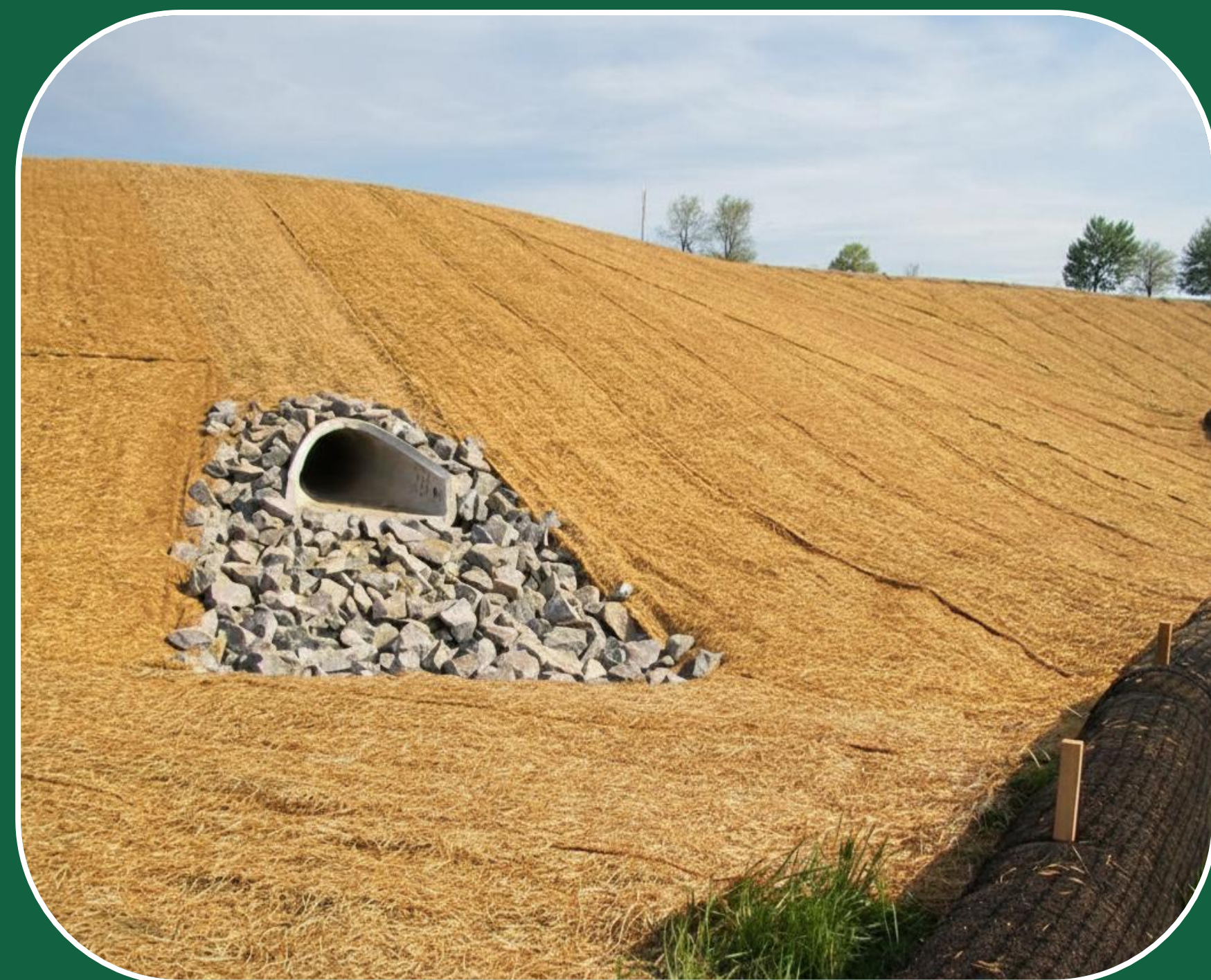
Erosion Protection Over New Roadway Embankments.
