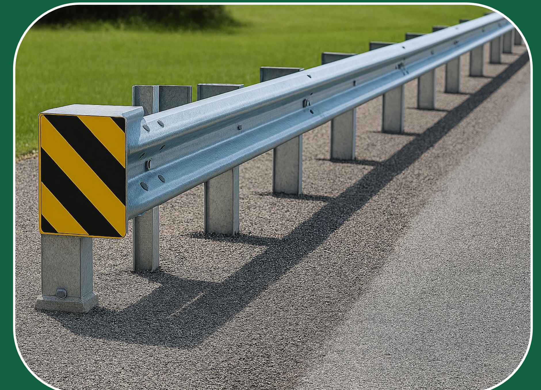
New Steel Beam Guiderail Along the Eastbound Lane.
