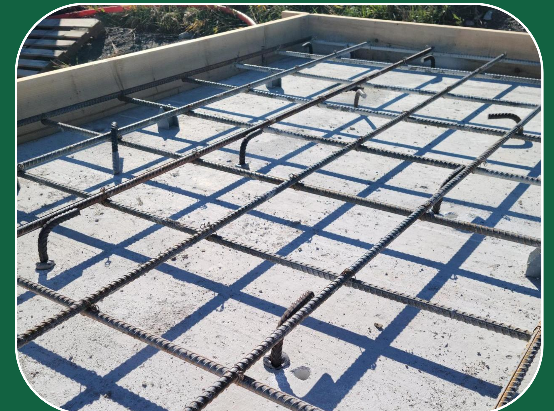
New Waterproofing and Distribution Slab on Tunnel to Prevent Water Infiltration.
