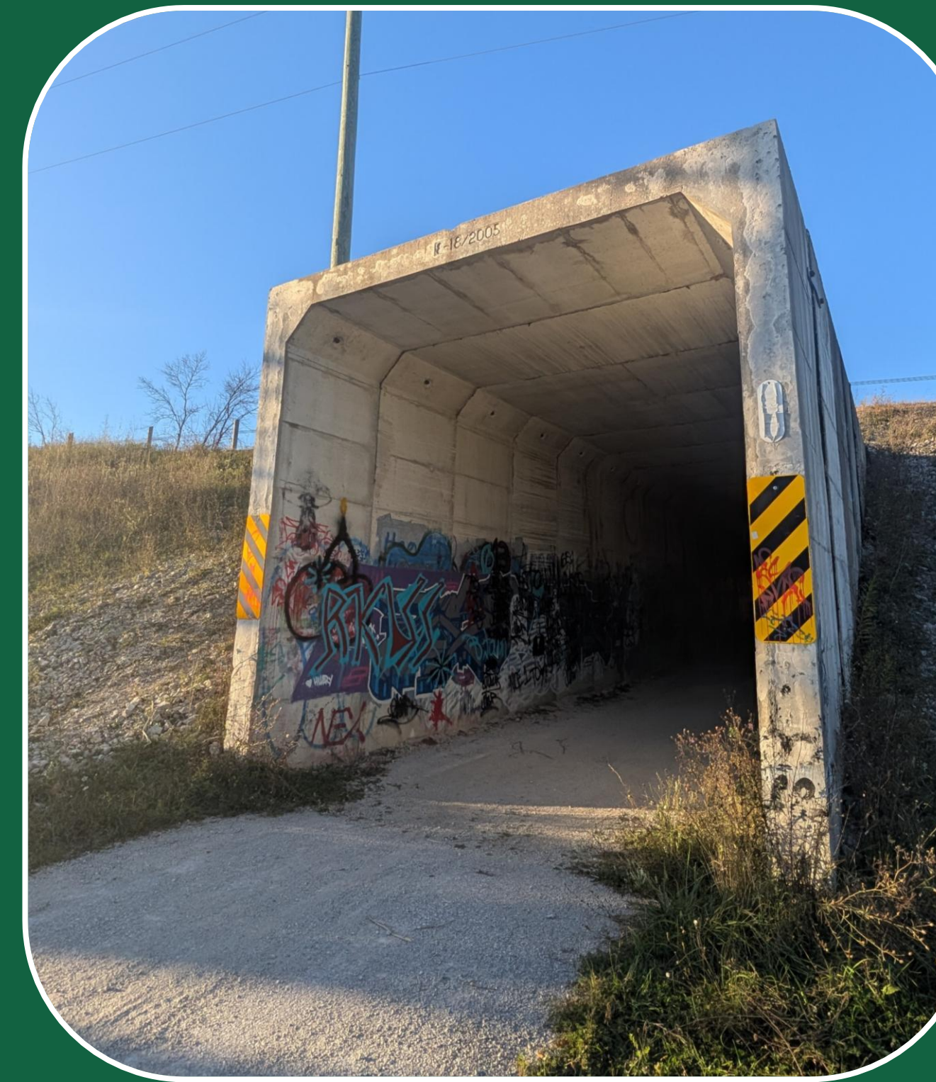
View of Structure Facing North.
