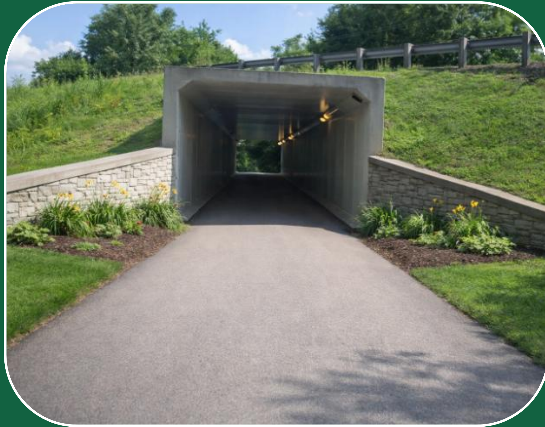
New Segmental Block Retaining Walls Beside the Tunnel.
