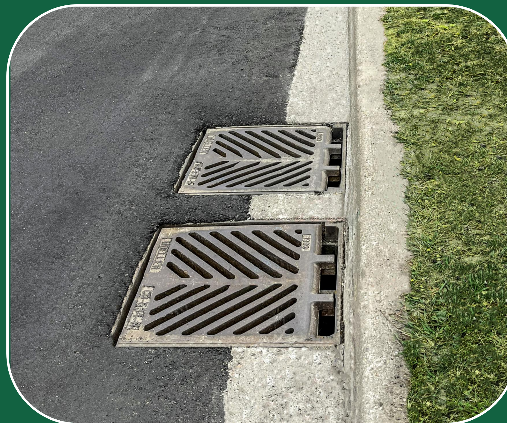
New Stormwater Catch Basins.
