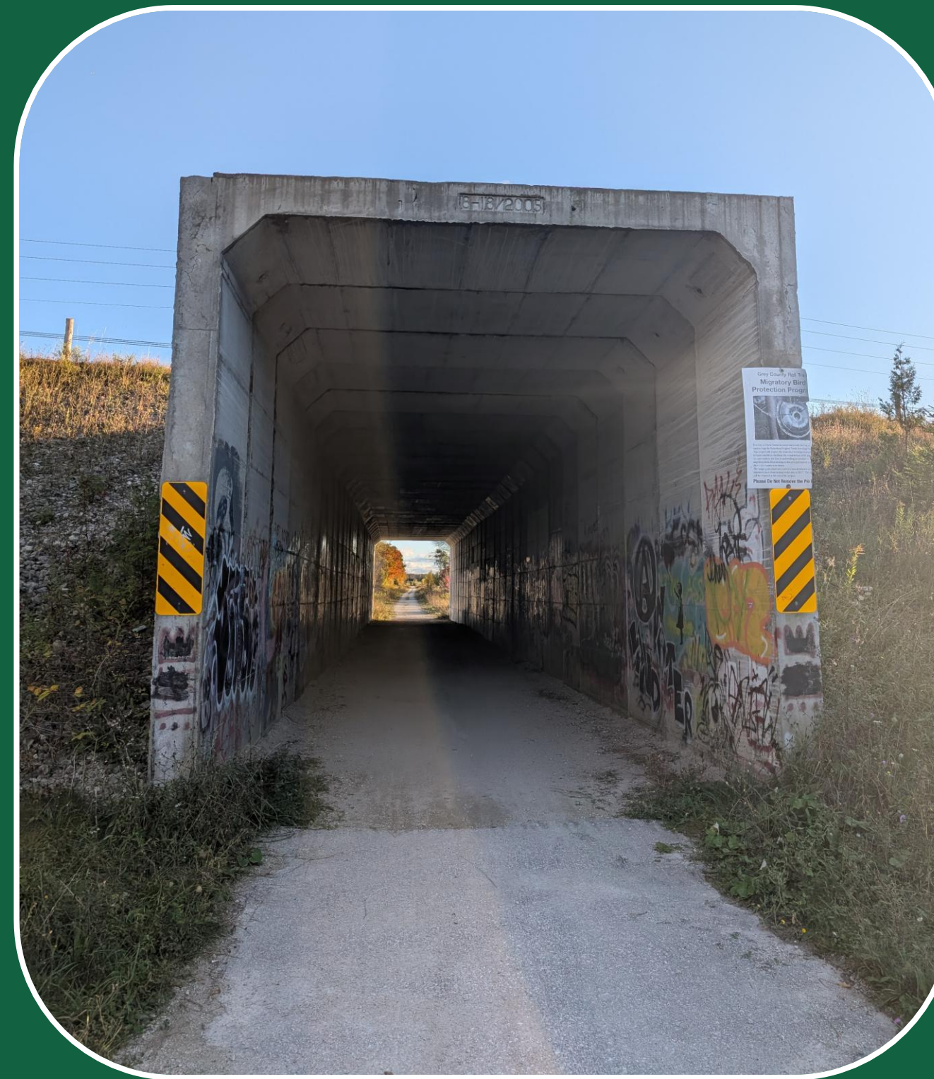
View of Structure Facing South.
