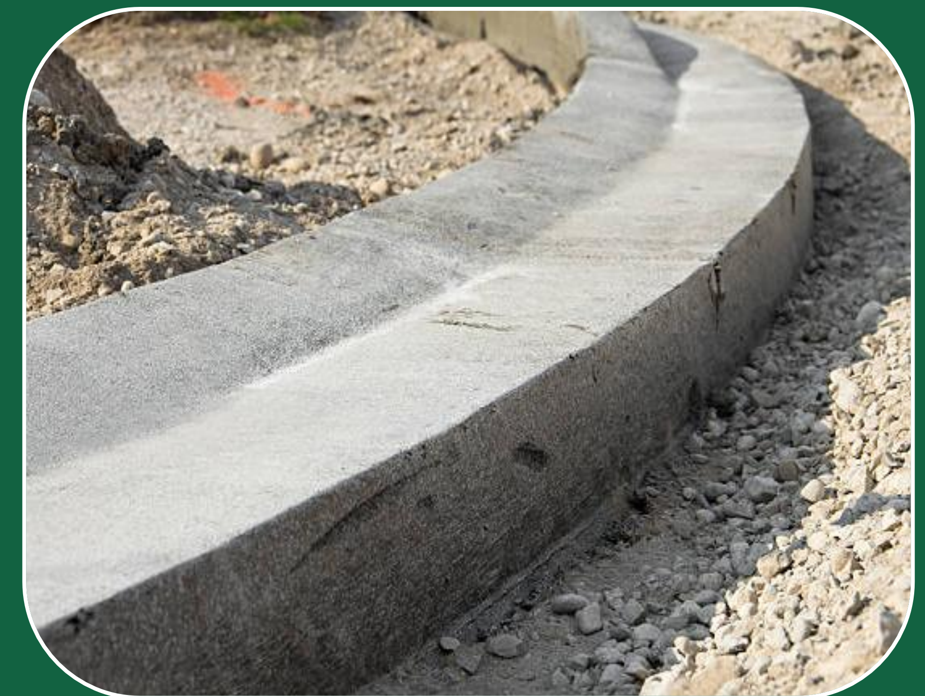
New Mountable Curb and Gutter Along the Eastbound Lane.
