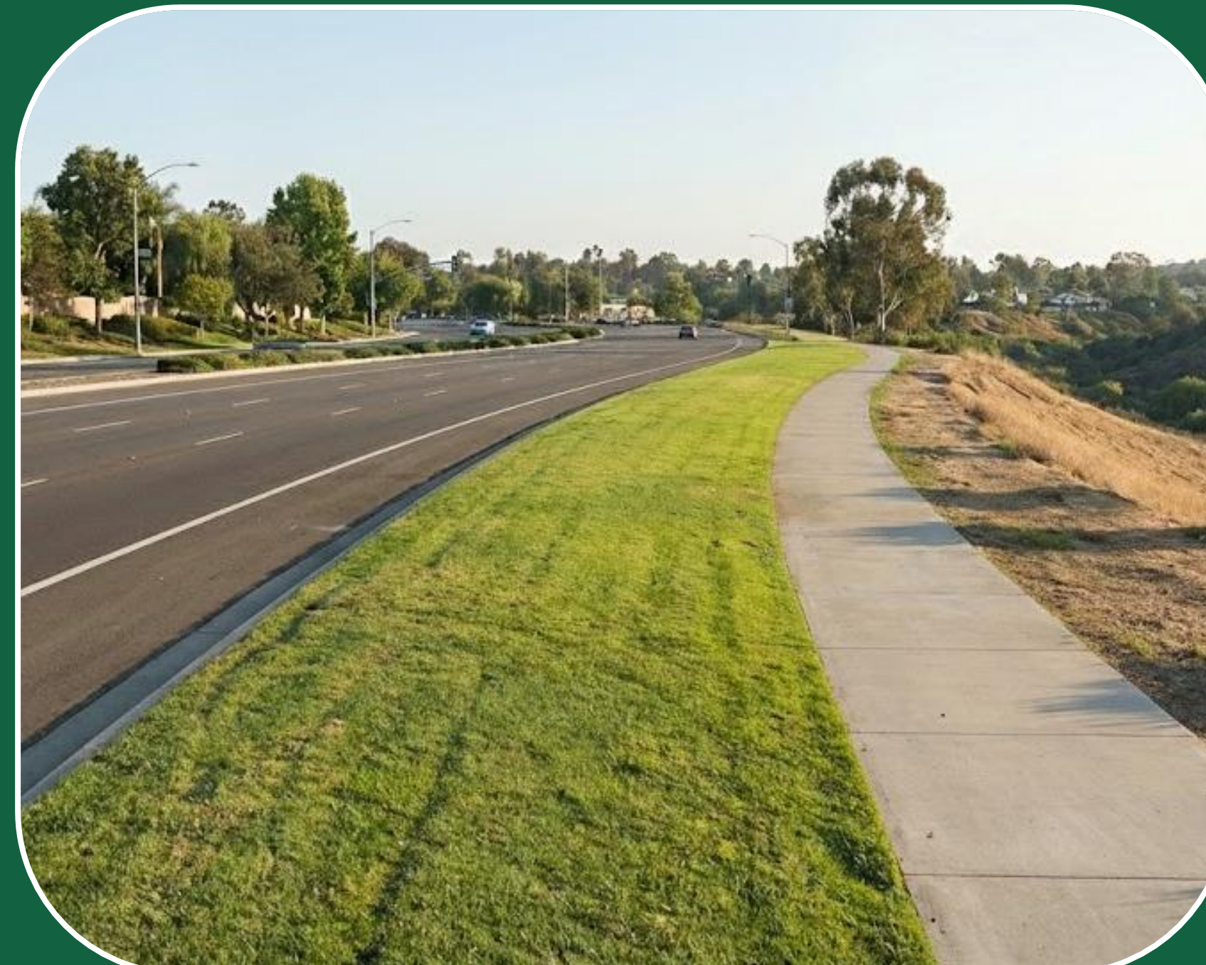
New Sidewalk Along the Eastbound Lane.
