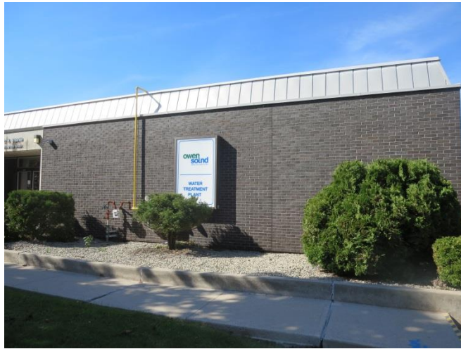
Richard H. Neath Water Treatment Plant
